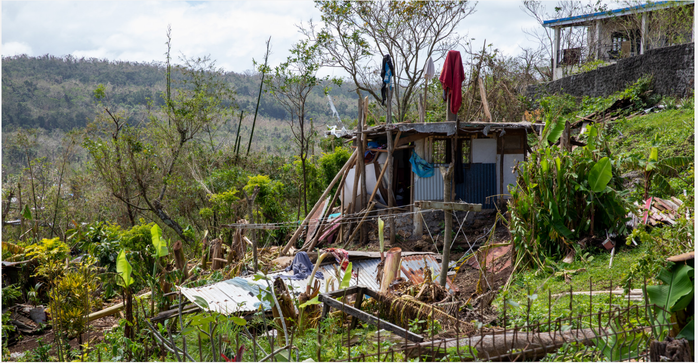
Twin Tropical Cyclones Judy and Kevin hit Vanuatu only 48 hours apart. Many homes were destroyed, leaving affected families seeking temporary shelter in evacuation centres and makeshift dwellings.
