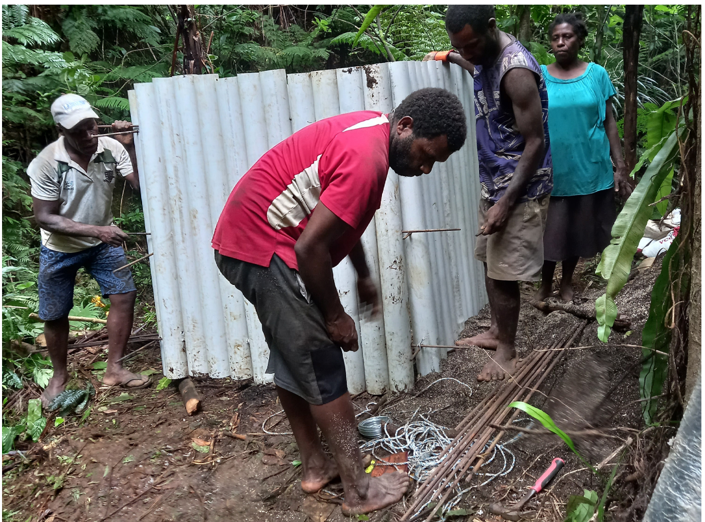
Community members set up a water catchment box ready to be installed in their village.
