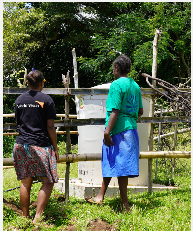
Linda shows Vanessa, a staff member from World Vision Vanuatu, the water tank that is part of the new system upgrade in her village.
